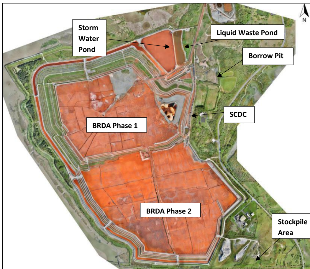
Figure 2.6: Aerial View of the Subject Site (Source: Golder, 2021 – Cropped and Annotated by Tom Phillips + Associates).
